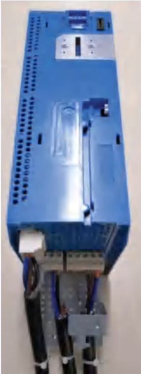
EMC wiring of Power Module B1
